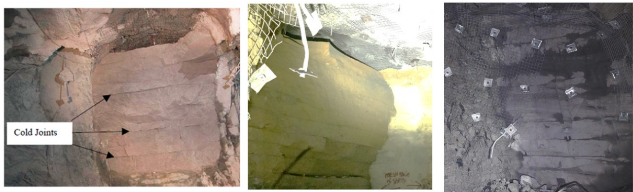
Figure 3. Cold/flow jointing in two different paste backfill masses.
