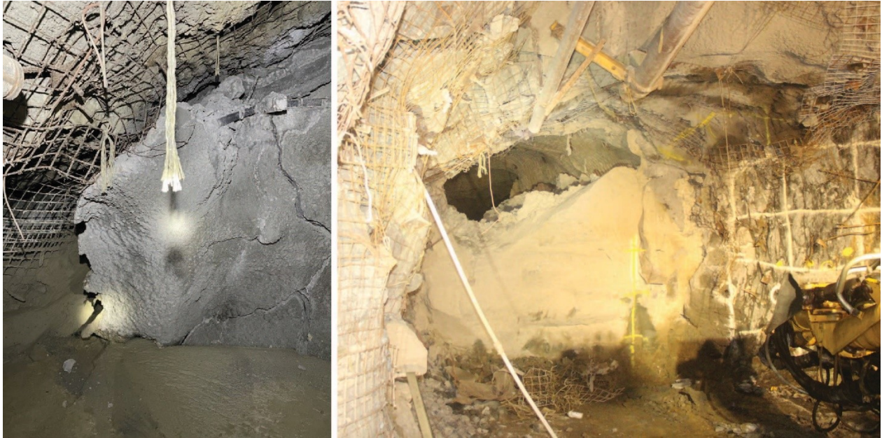
Figure 5. Images of the displaced barricade which was subsequently partially dismantled to reveal paste above the 3/4 barricade height had been discharged either during the original displacement, or the subsequent extensive flushing.
