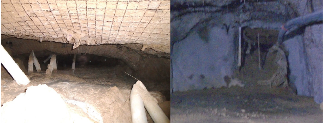
Figure 2. View within the drift showing volume of remnant backfill and bent breather pipes (left); the barricade failed on one side (right).
