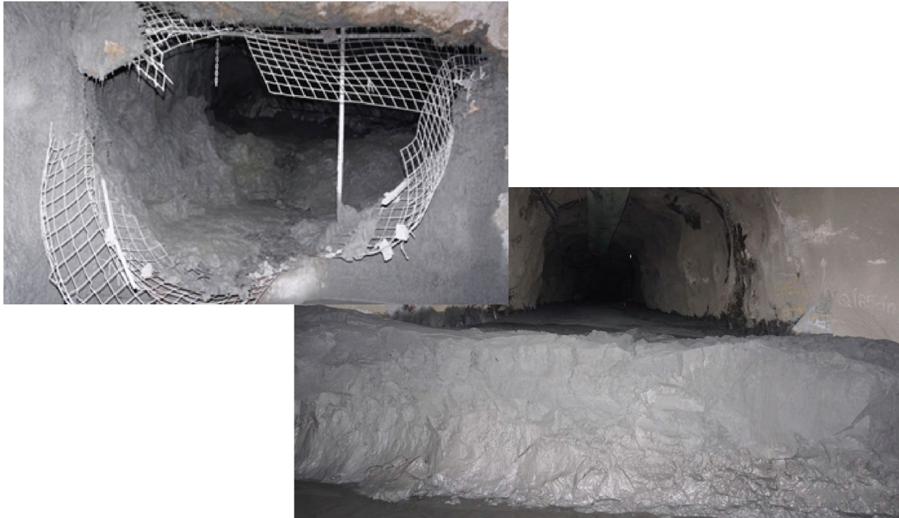
Figure 6. Failed barricade and paste excavated from intersecting drift an estimated 100 m from the barricade (From Gray, 2019).
