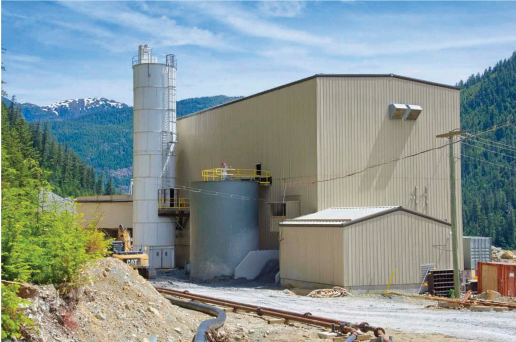
Figure 11. Paste plant building complete with new binder silo and filter feed tank.
