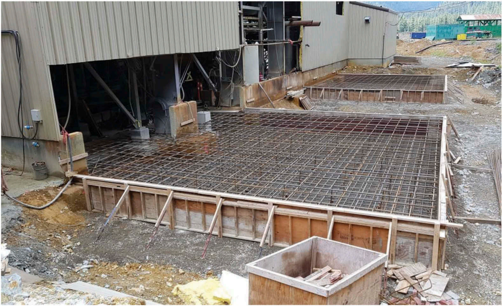
Figure 8. Silo and filter feed tank raft footings.
