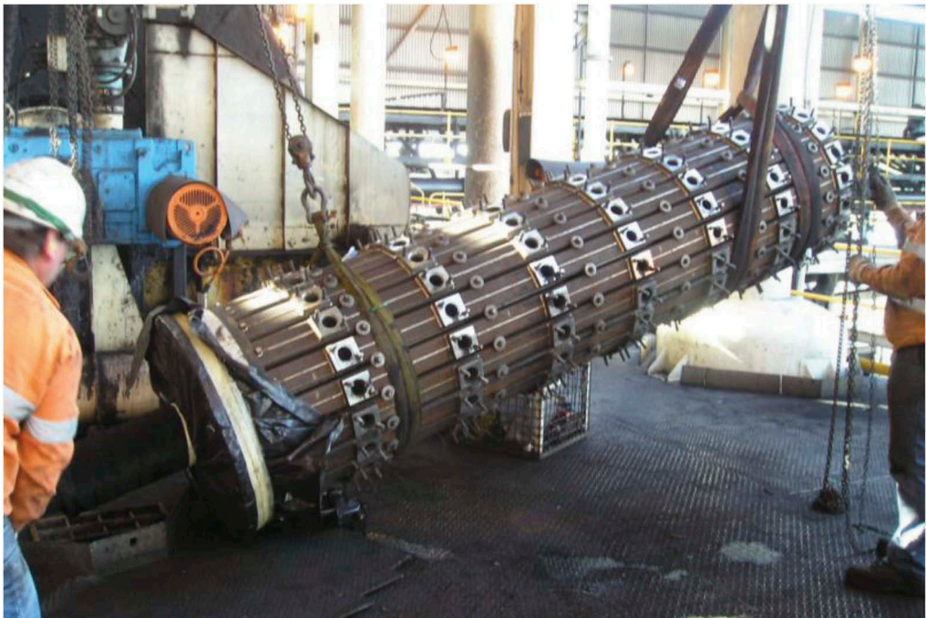
Figure 6. Lifting of new filter barrel.
