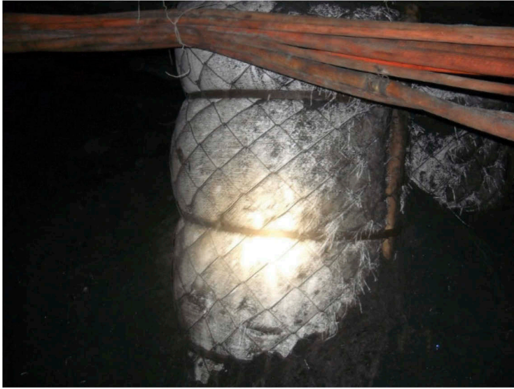
Figure 2. Circular grout pack with steel reinforced cage.
