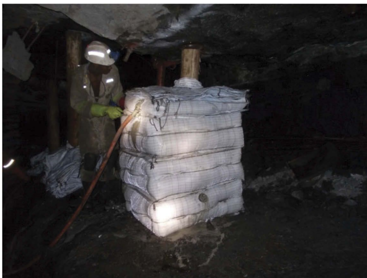
Figure 1. Square grout pack.
