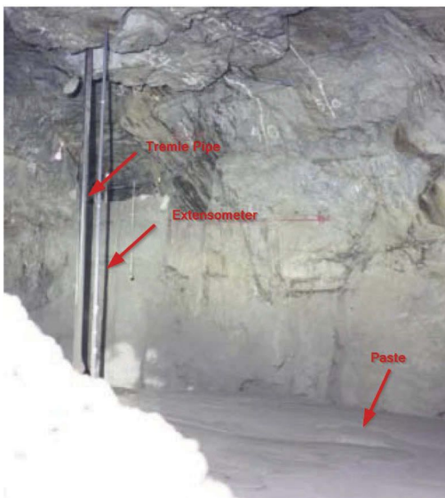
Figure 7. Image of the tremie pipe and extensometer taken with underground camera. Source: Nahami Construction Limited underground camera record.
