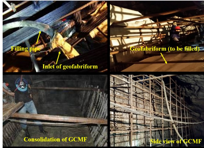
Figure 10. GCMF filling and consolidation.
