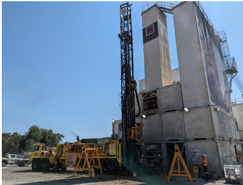
Figure 6. Epiroc RD20 drill rig swapping out mines' surface borehole pipe.
