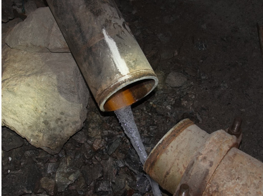
Figure 3. Unpiped borehole with significant water ingress flowing through piping.
