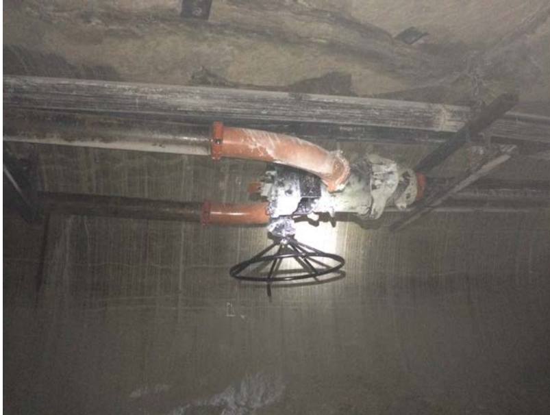
Figure 3. Victaulic Series 725 Diverter Valve installation
