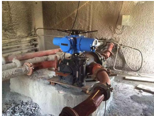
Figure 7. Electric actuator application install
