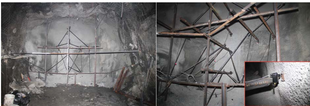
Figure 4. View of the displacement array frame positioned in front of (but not in contact with) the shotcrete barricade. The insert shows a potentiometer attached to strut extending from the frame.
