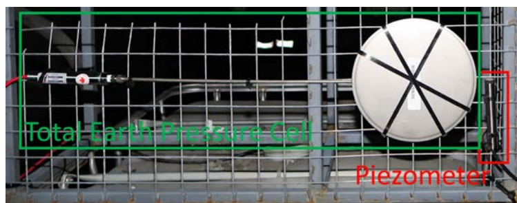
Figure 4. Total earth pressure cell and piezometer used in the installation
